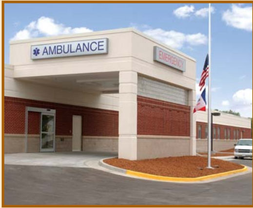
Emergency Department entrance at Marengo Memorial Hospital
